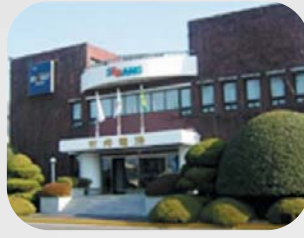
Chang-Won Factory Industrial battery & Motive Power, EV(Electric Vehicle) - Capacity : 1.5 Million/year - Gross Area : 28,000 m 2
